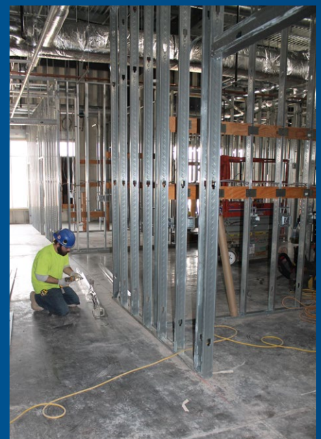
In February, the building's steel studs were up.
